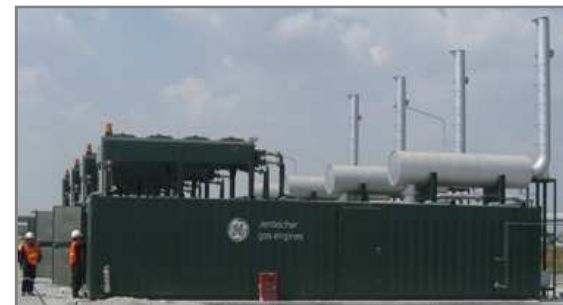
Electricity generated using GE 320 1063KW biogas engines
