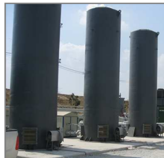
Gas not required for generation is flared
