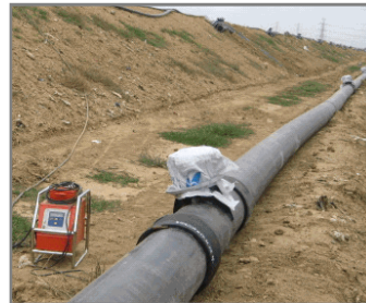
Collected landfill gas transported via carrier pipes to generation compound
