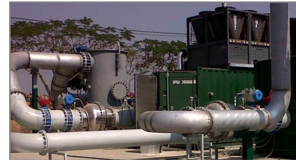
Landfill Gas enters pre-treatment plant
