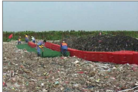
Installation of gas collection pipes
