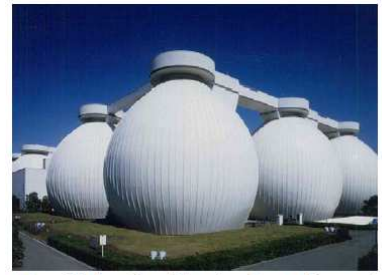
Raw Sludge Gas Digester Power Generator (Yokohama facility)
